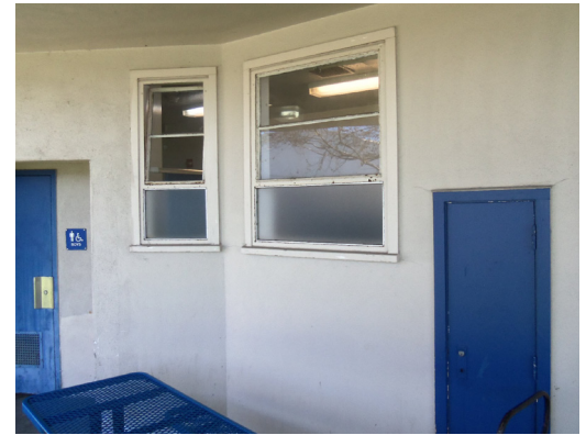
Door hardware is non-ADA compliant and window systems need replacement at Culver City High School cafeteria building.
